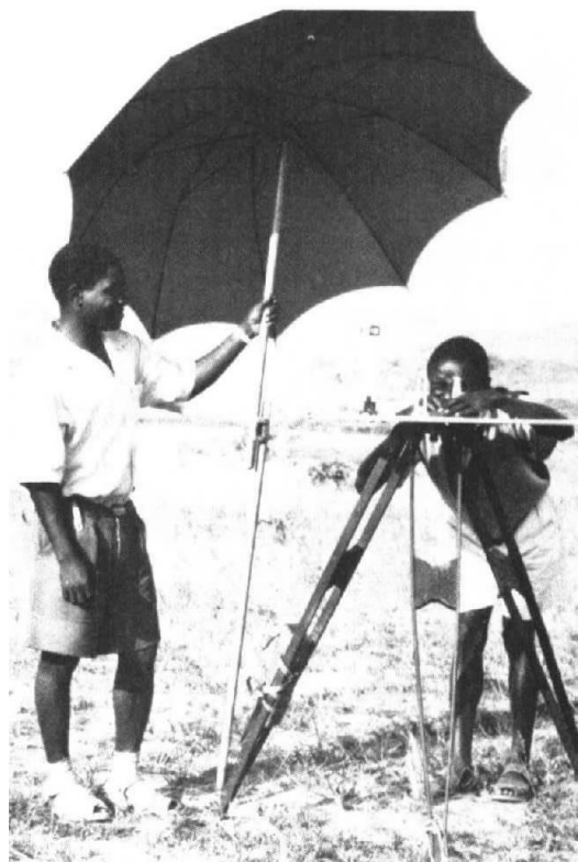
Survey team for road construction Courtesy Embassy of Nigeria, Washington
