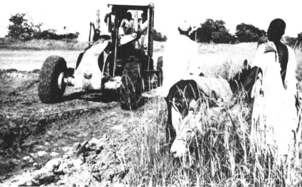
Preparations for building bridge over Gongola River, an infrastructure development project Courtesy World Bank
